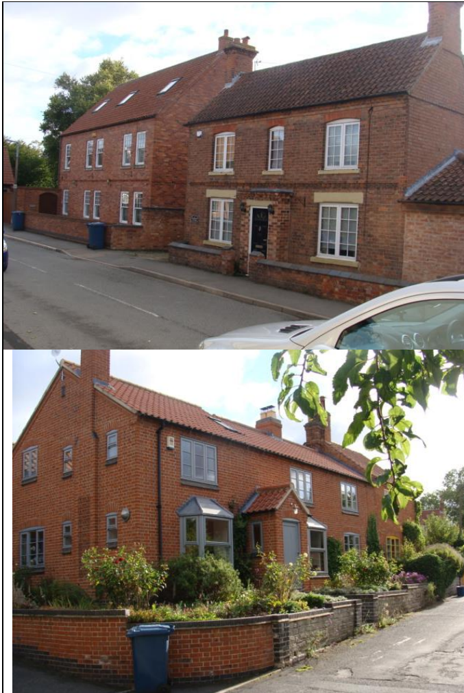
There are examples of sensitively designed new buildings within the conservation area
